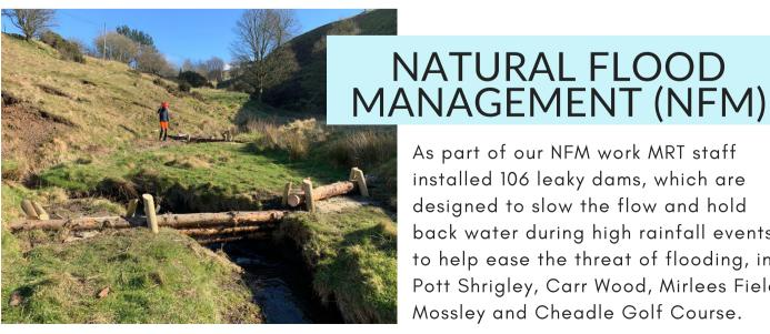
As part of our NFM work MRT staff installed 106 leaky dams, which are designed to slow the flow and hold back water during high rainfall events to help ease the threat of flooding, in Pott Shrigley, Carr Wood, Mirlees Field, Mossley and Cheadle Golf Course.
