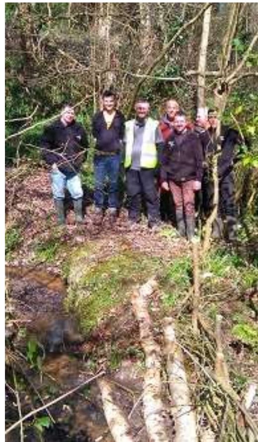
Fig 8. Volunteers installing Leaky Dams at Rivacre Brook
